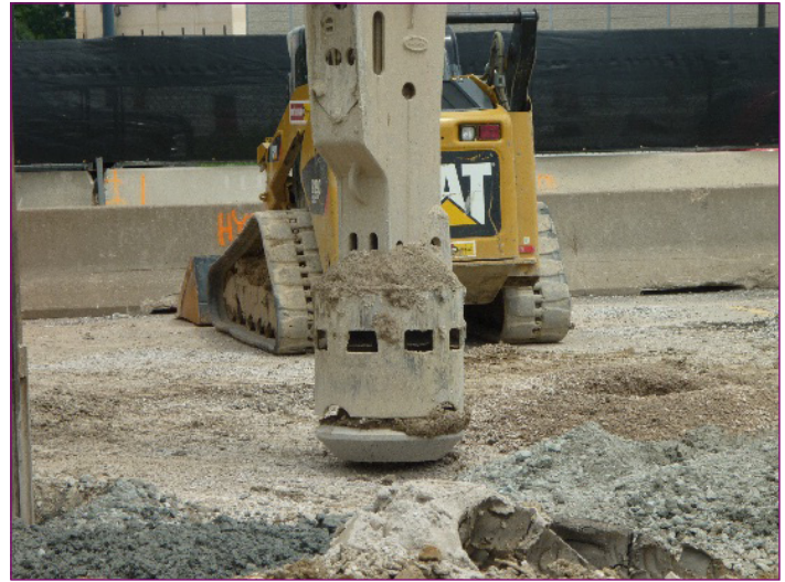
Figure 3: Bevelled tamper increases lateral pressure.
