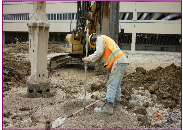
Figure 5: Conducting the Dynamic Cone Penetrometer Test (DCPT) with hand-held equipment.
