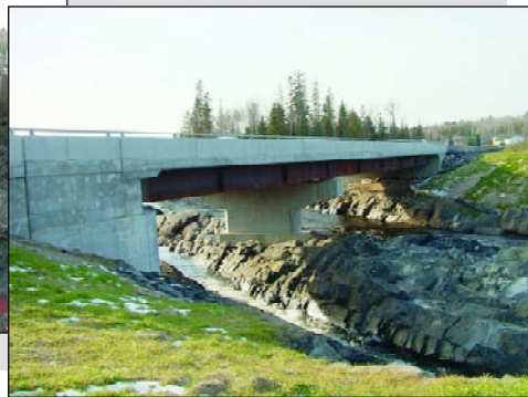
Highway 144 project "after"
