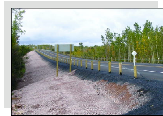
Highway 11/17 project "after"
