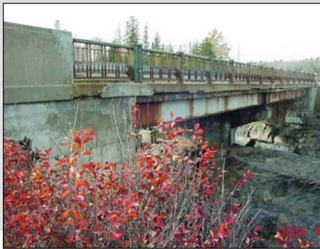
Highway 144 project "before"
